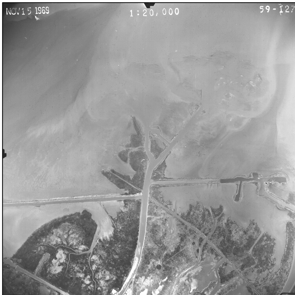
15 November 1969: Prior to Baptiste Collette channel construction
